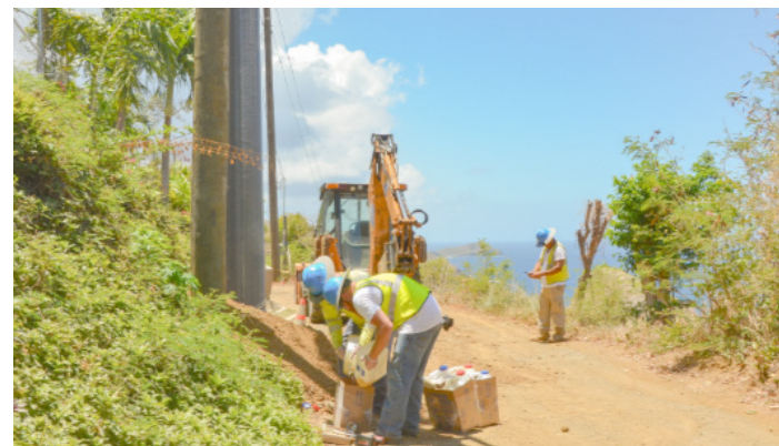
Haugland Energy Group installs composite poles on St. Thomas.
