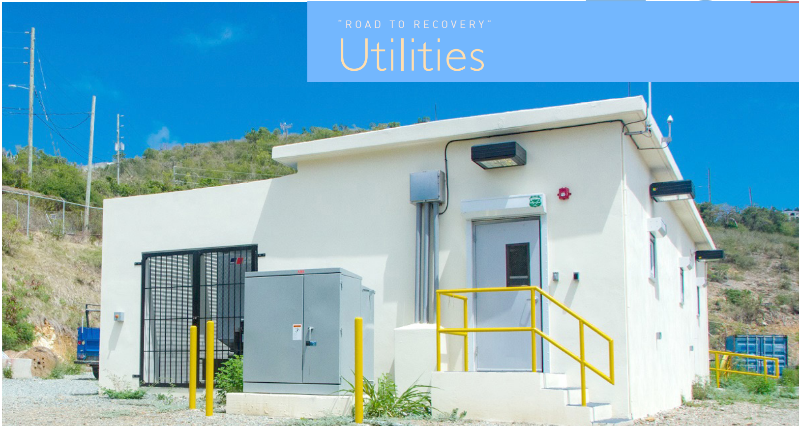
East End Electrical Substation on St. Thomas
