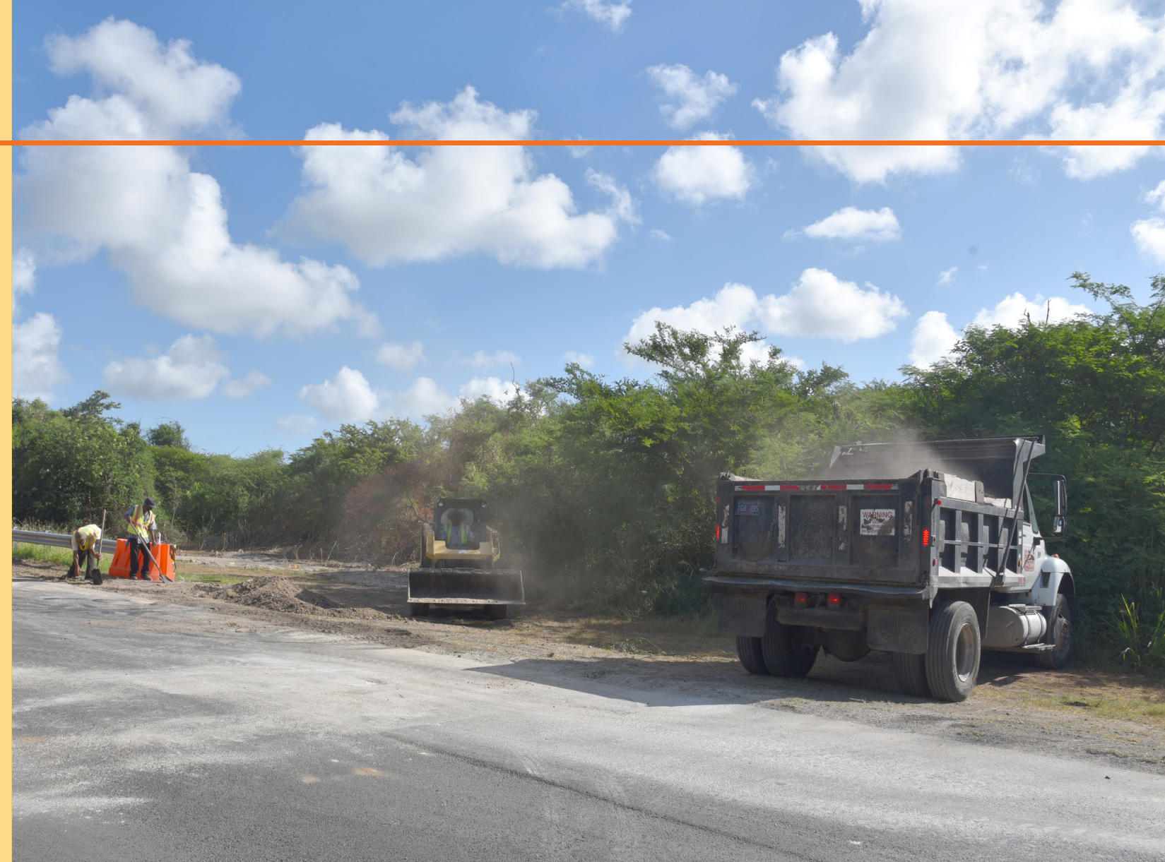
Construction at East Airport Road on the Melvin Evans Highway
