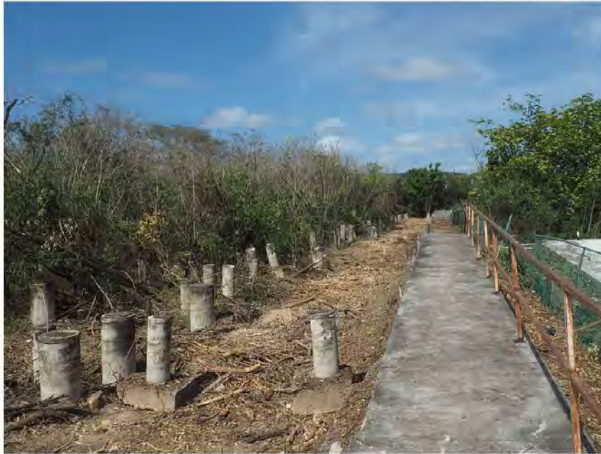
Figure 2. Sidewalk, Pilings, and Secondary Forest.
