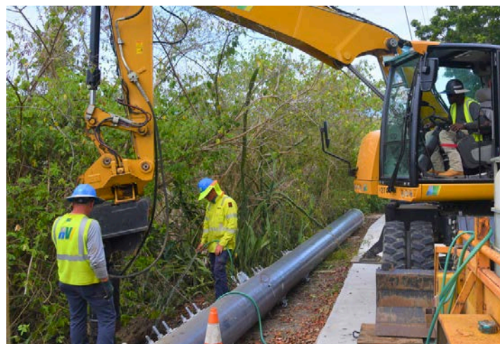
Composite Pole Installation on St. Croix
